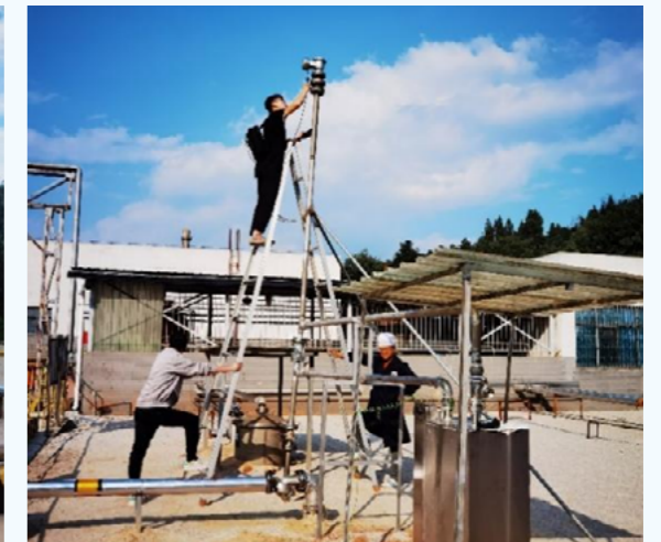
Renovation at the End of Breathing Port of N-hexane Storage Tank in Qidian Industrial Zone
